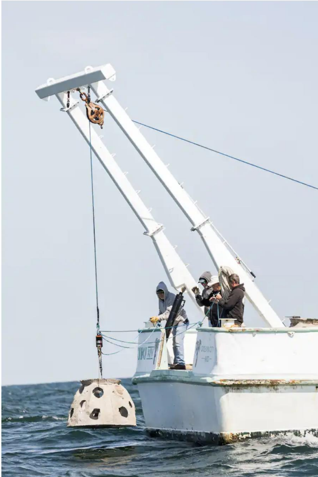
A crane lowers a reef ball into the water. (Tiffany Caldwell/for The Washington Post)
